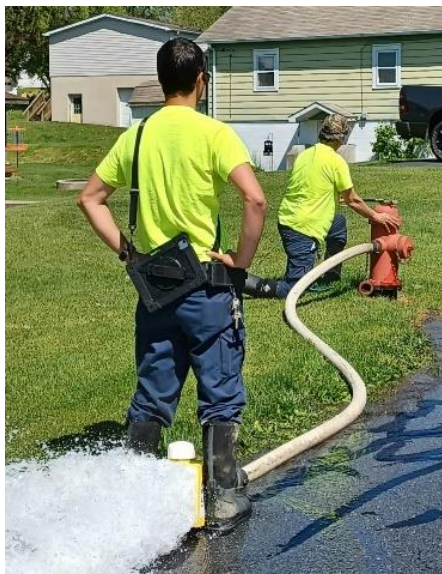
Hydrant Flushing
